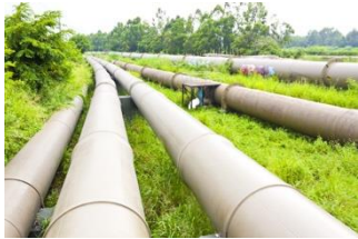
Infrastructure and Environment
